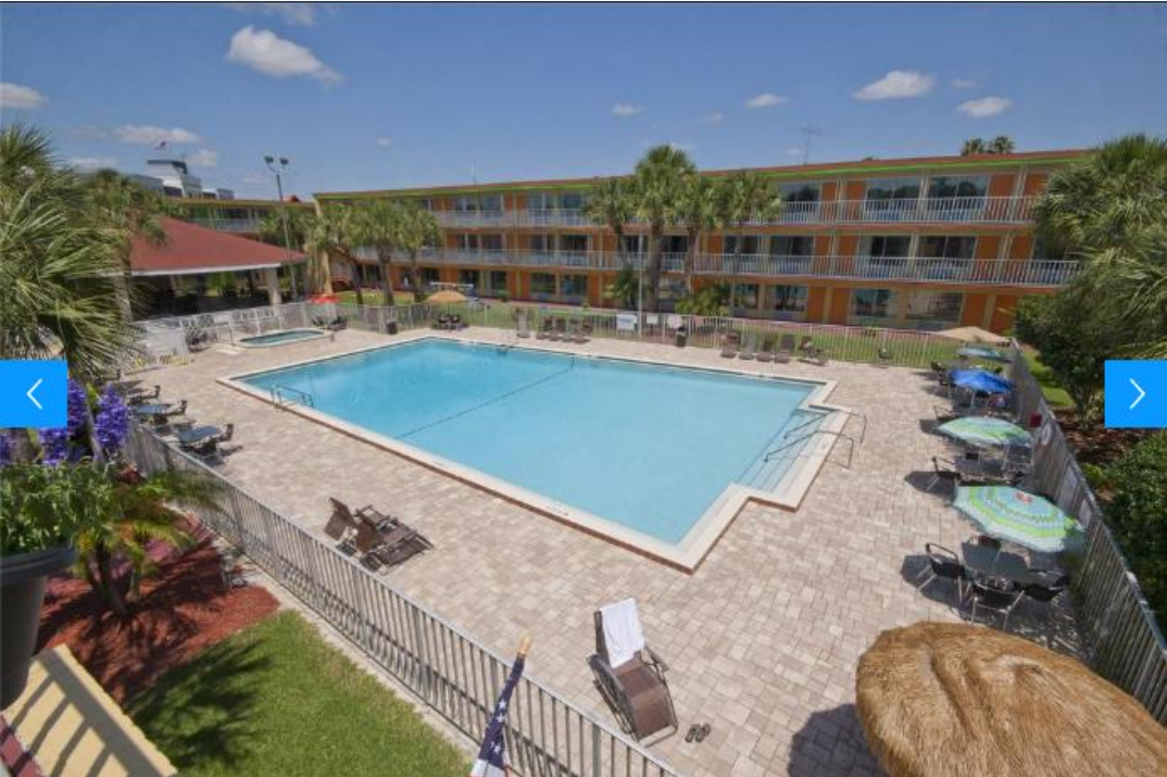
Roomba Inn Orlando
